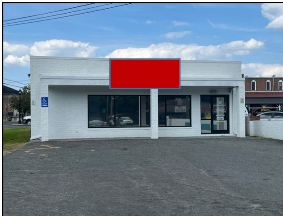
6605 E. Marshville Blvd. (Achievement Center) Actual façade size: 468 sq. ft. Illustrated sign size: 47 sq. ft. (10% of façade)
