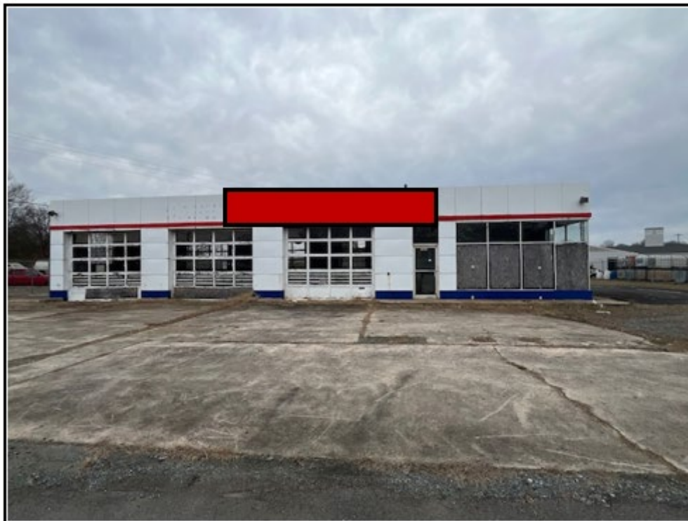
Subject property: 6349 W. Marshville Hwy. (old Cooper Tire/Amoco site) Façade size: 1,008 square feet Depicted sign size: 101 square feet (10 percent of façade size)
