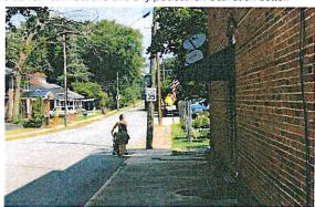
3) Looking north on N Elm Street, showing ADA compliance issues including a lack of curb ramps, tactile warning strips, and minimum sidewalk width around obstructions (utility poles)
