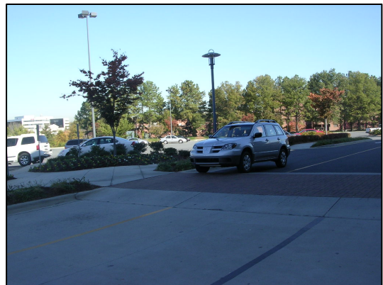
A raised crosswalk connecting a parking lot to a storefront, but lacking paint markings that would increase visibility
